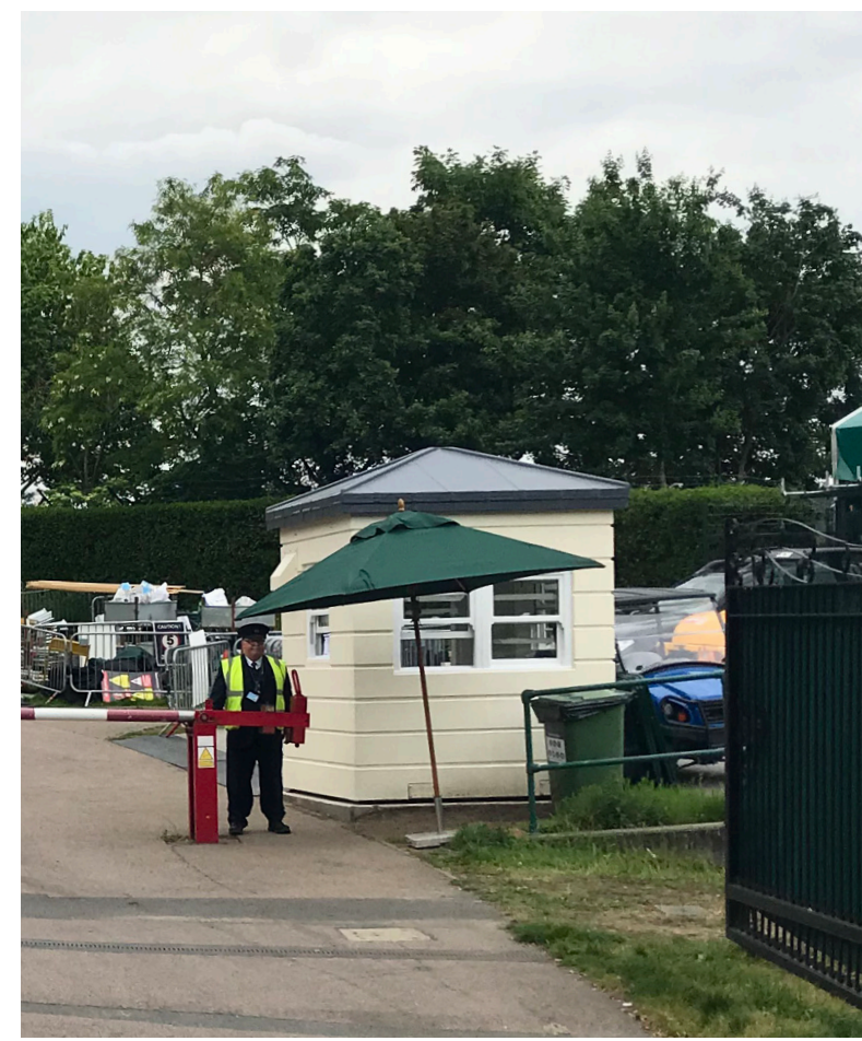
Existing Security Gatehouse 1
